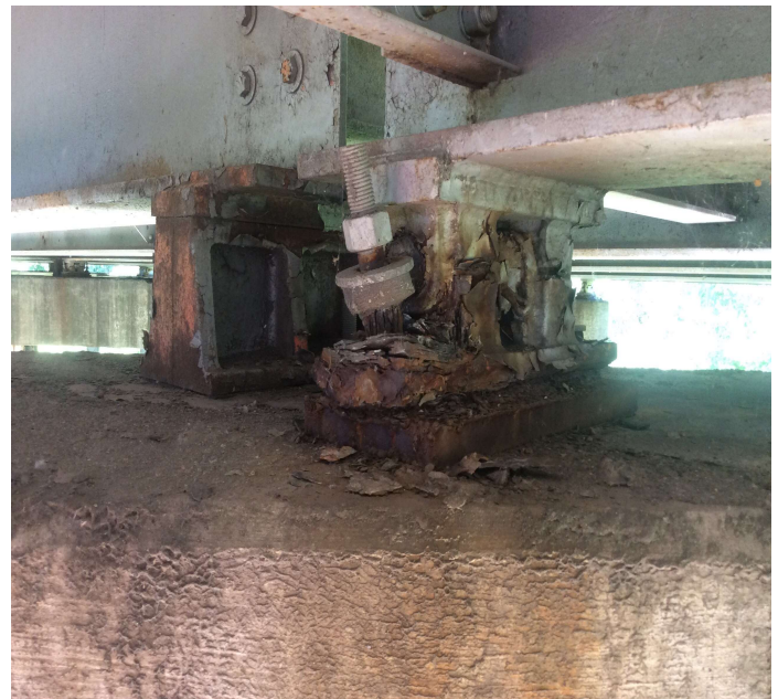
PHOTO 2 Description Bent 8 moveable bearing 6 has pack rust. Typical condition.
