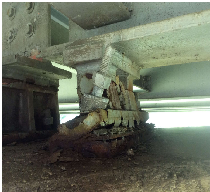
PHOTO 1 Description Most all bearings have pack rust.
