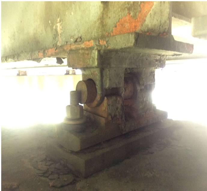
PHOTO 1 Description Bent 6 span 6 beam 3 bearing pin is working out and moving under traffic.
