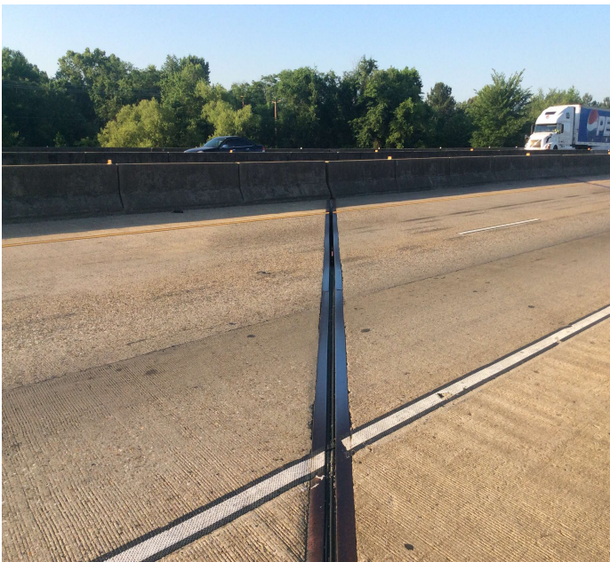
PHOTO 1 Description Bent 3 has 20' joint material that has fallen out.
