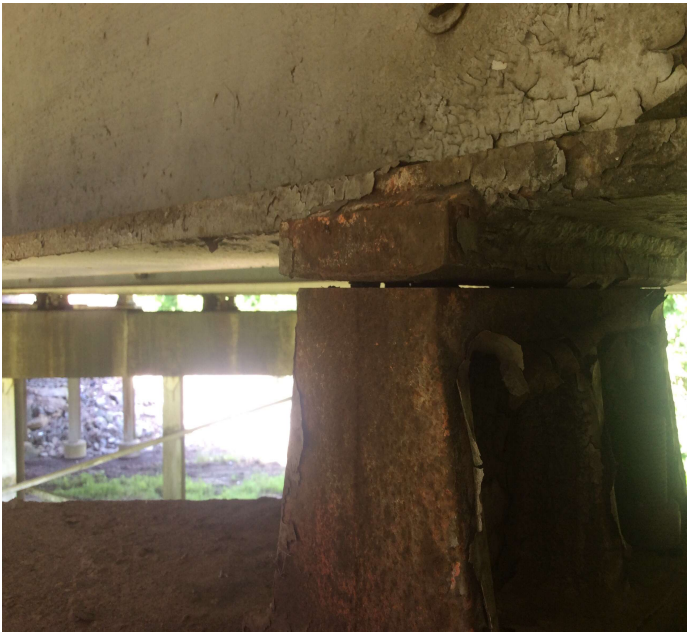
PHOTO 1 Description Bent 3 fixed bearing 4 has movement under traffic impact.
