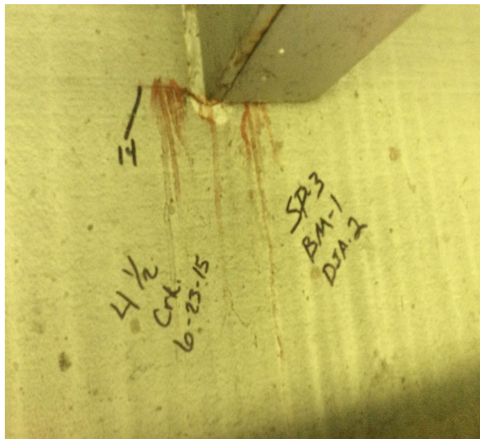
PHOTO 1 Description 4 1/2 inch crack span 3 beam 1 dia. 2 at bottom of dia. Bracket.
