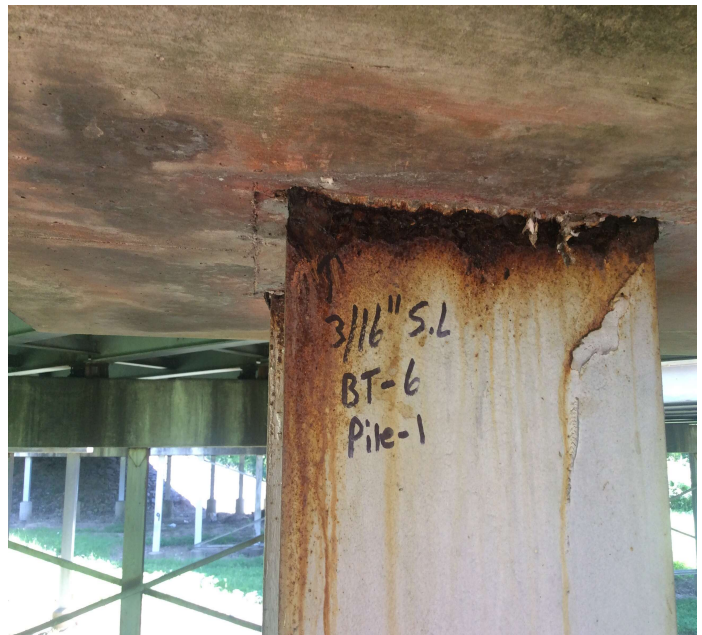
PHOTO 2 Description Bent 6 pile 1 has 3/16\" section loss in top of pile.
