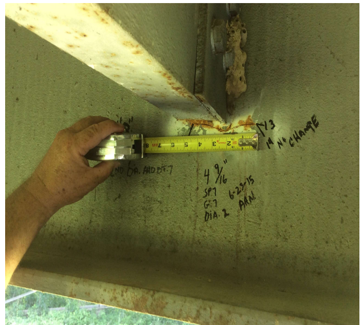
PHOTO 2 Description Span 7 GDR 7 second diaphragm. Has a 4 9/16 inch long crack in web at bottom of diaphragm bracket.
