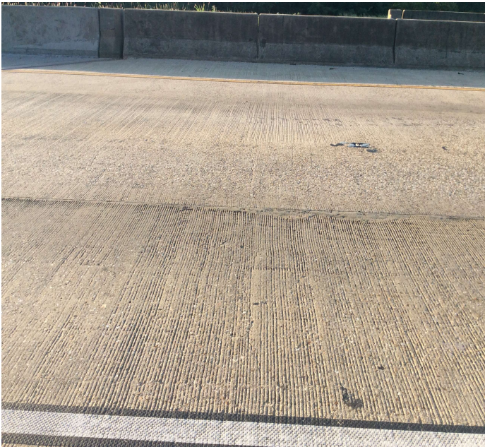
PHOTO 1 Description Span 10 large transverse cracks.
