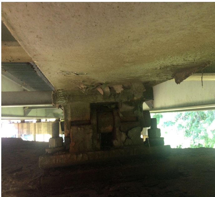
PHOTO 3 Description Bent 6 moveable bearing 3, bearing pin is working out.
