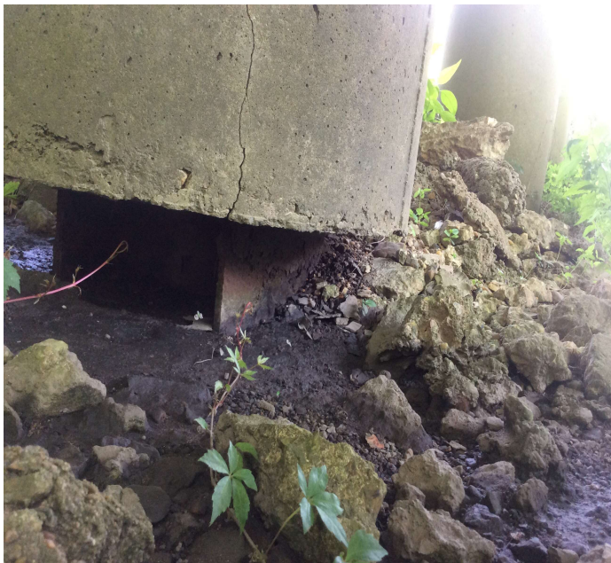
PHOTO 1 Description Erosion or scour has undermined concrete encasement exposing steel piles at ground level.
