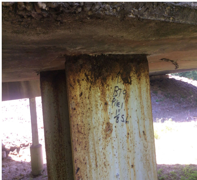
PHOTO 3 Description Bent 9 steel pile 1 has up to 1/8" section loss at the top.
