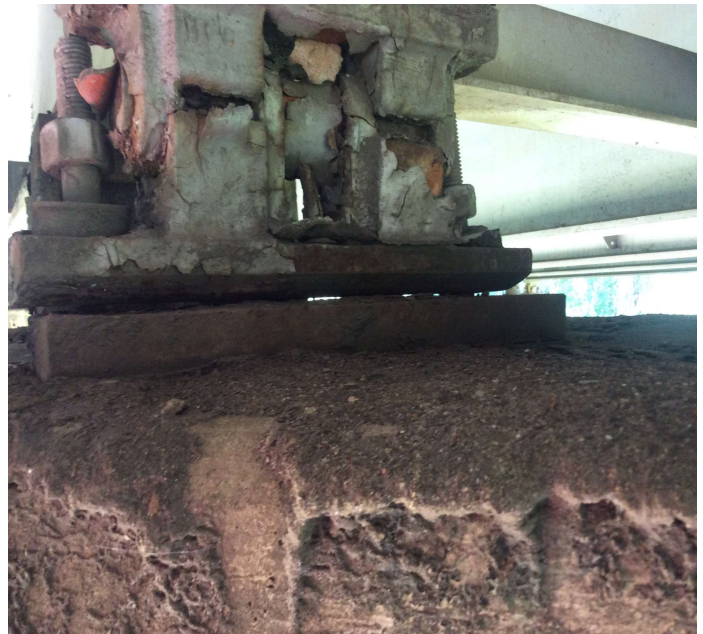
PHOTO 2 Description Bent 6 moveable bearings 5 and 6 have up to 3/8" movement when under traffic impact.
